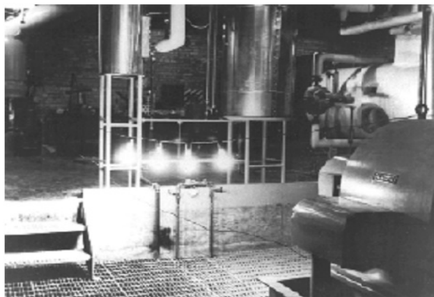
The Experimental Breeder Reactor I generated electricity to light four 200-watt bulbs on December 20, 1951. This milestone symbolized the beginning of the nuclear power industry.
